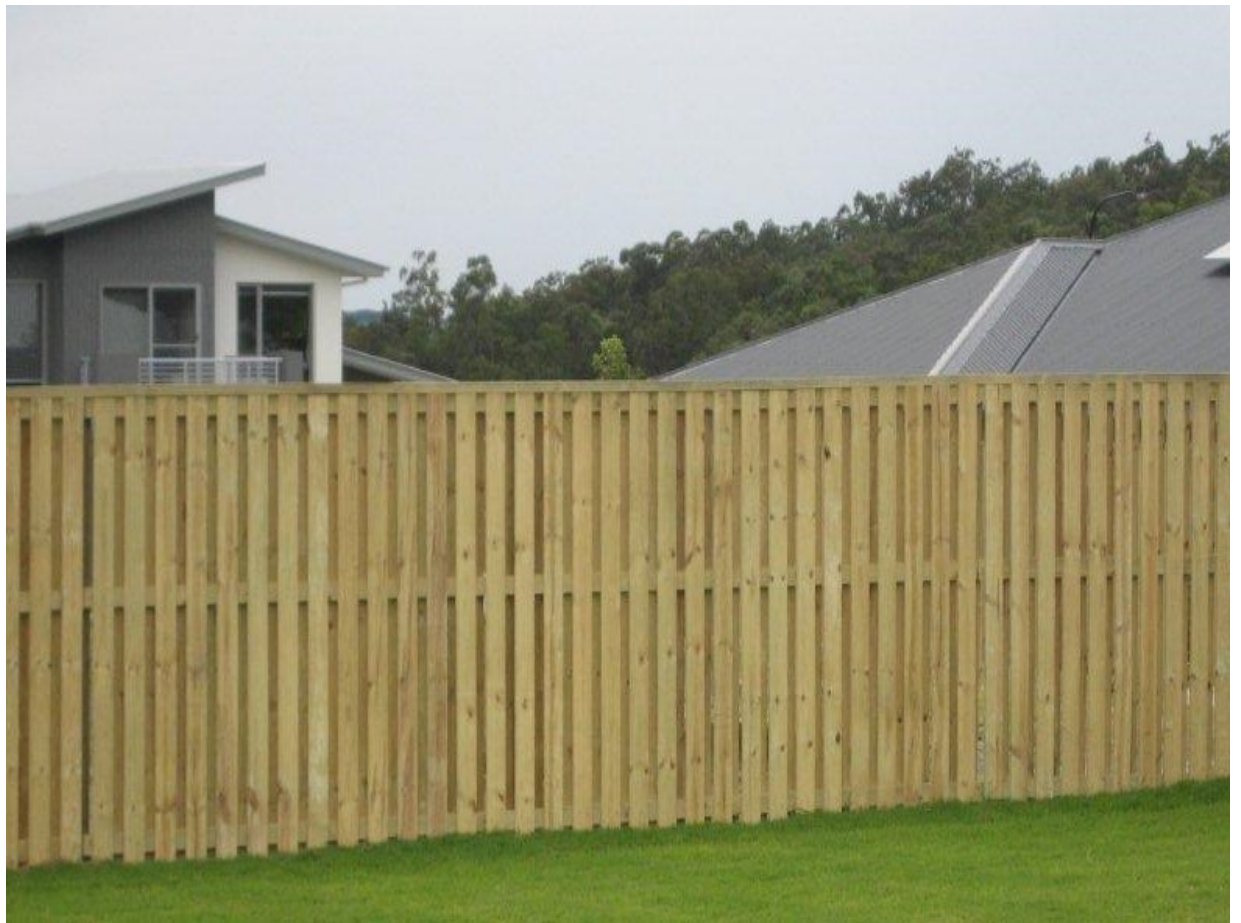
LAPPED AND CAPPED 1800 mm HIGH TIMBER FENCING
